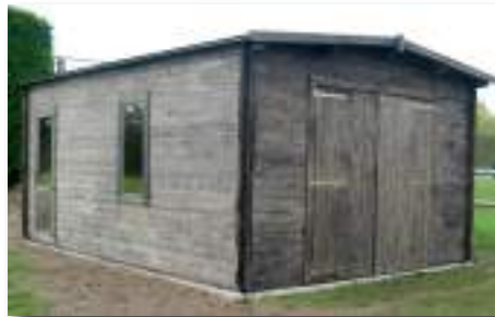
The new storage unit for the football club at Westwood Park, ready to be painted to match the pavilion
