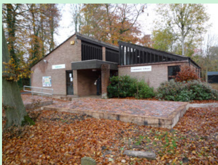
The library frontage is currently being landscaped
